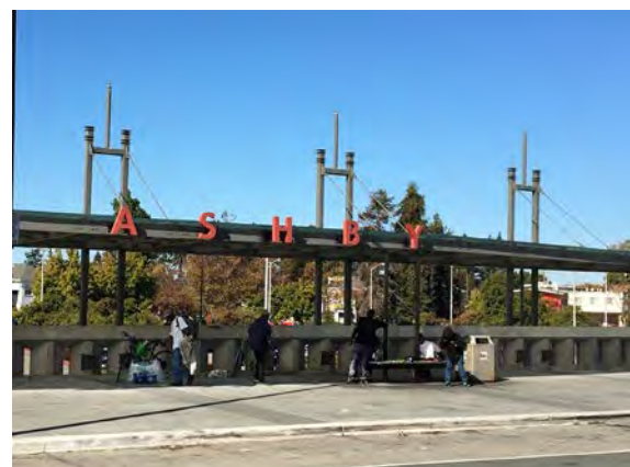
The Ashby BART Station
